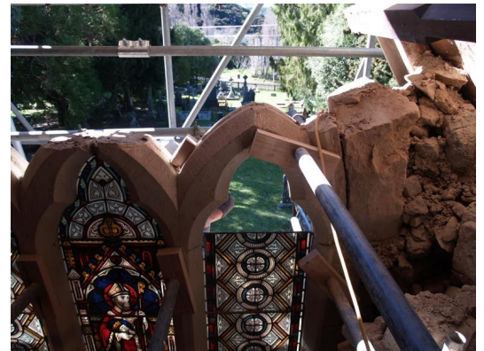
St Cuthbert's Church, Governors Bay had to be stabilized and the stone wall carefully removed by Ben West of StoneWorks to allow the safe removal of the window.
