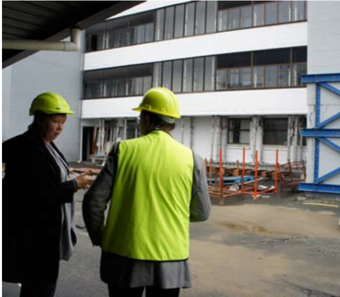
Alison explains the damage to the Bishopspark apartment building.
